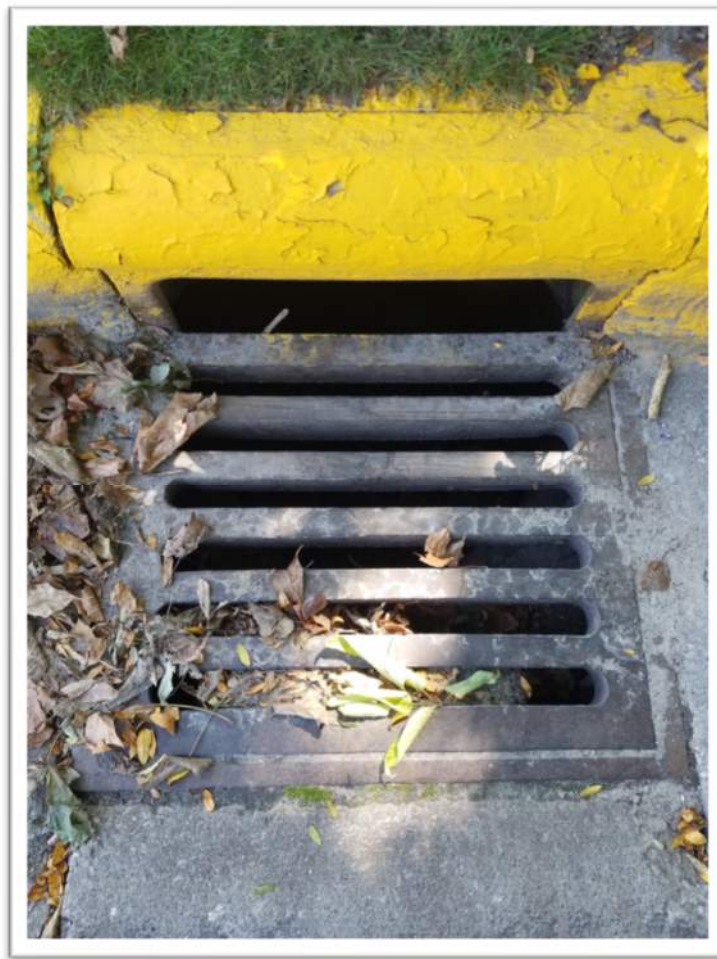
Exhibit 6 – Undersized Openings on the Catch Basins
