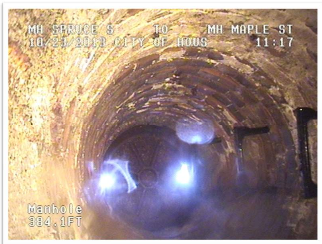
Exhibit 8 – Brick Sanitary Sewer Manhole Main at Maple Street
