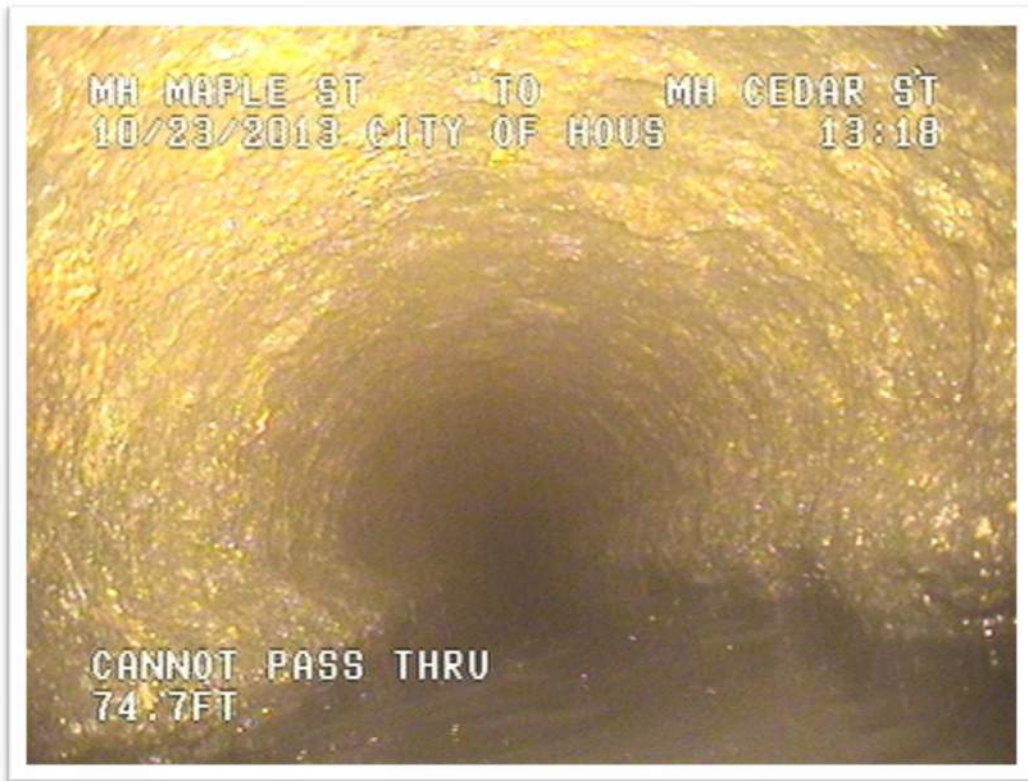
Exhibit 7 – Cast Iron Sanitary Sewer Main Obstructed 75-ft North of Maple Street
